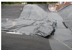
Re-lining of Scott's Mill
