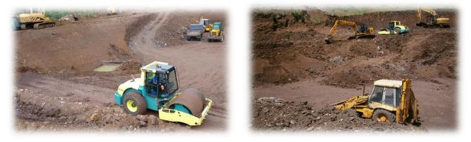
Although excavating a bigger hole in the ground appears easy, it requires sound engineering to ensure the end result will meet the objective of increased storage and improved water security. Every stage during construction will be carefully monitored, works properly measured and compaction tests being carried out to ensure built strength and
