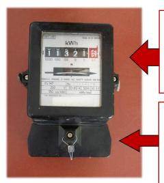
Damage to screws or fixings may indicate a loose cover. Live wires could be exposed.
