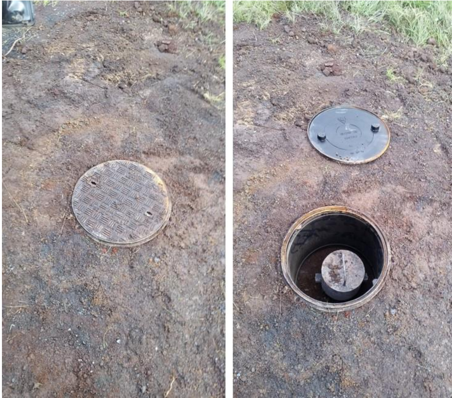
Figure 6: Example of completed borehole with a manhole and cover (Rosemary Plain)
