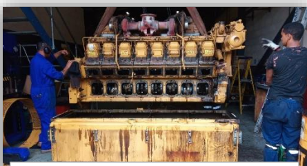
Lifting the engine block from the sump
