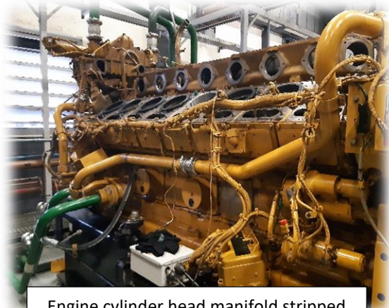
Engine cylinder head manifold stripped and cylinder head units taken out
