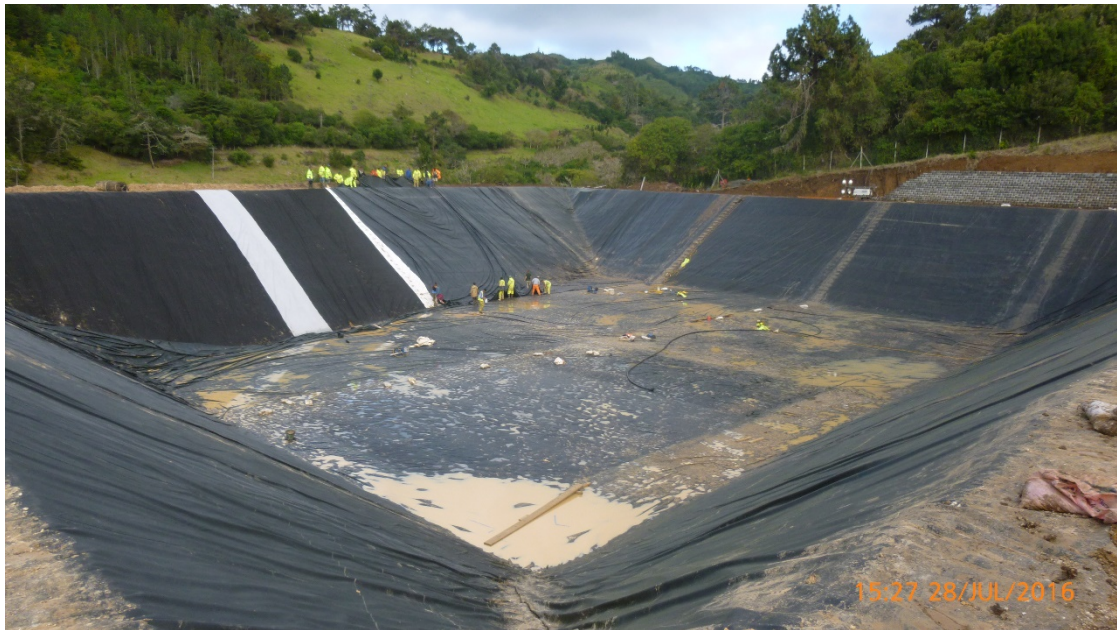
This photograph was taken during the lining of Harpers 3 reservoir
